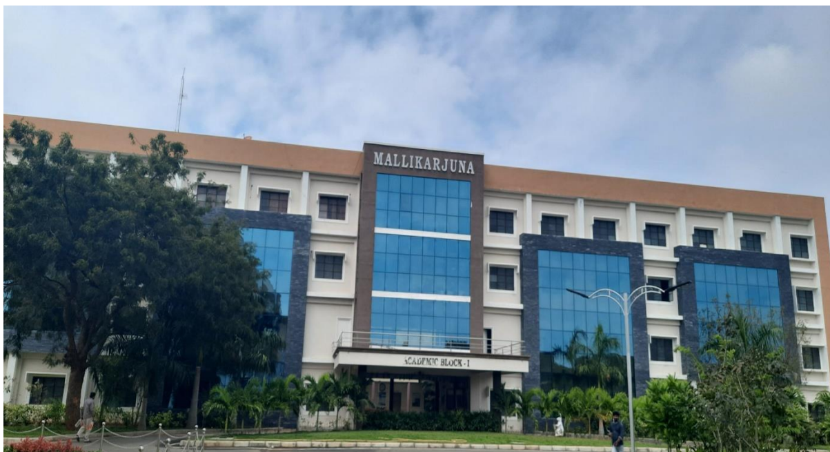
LED lights front of the Building
