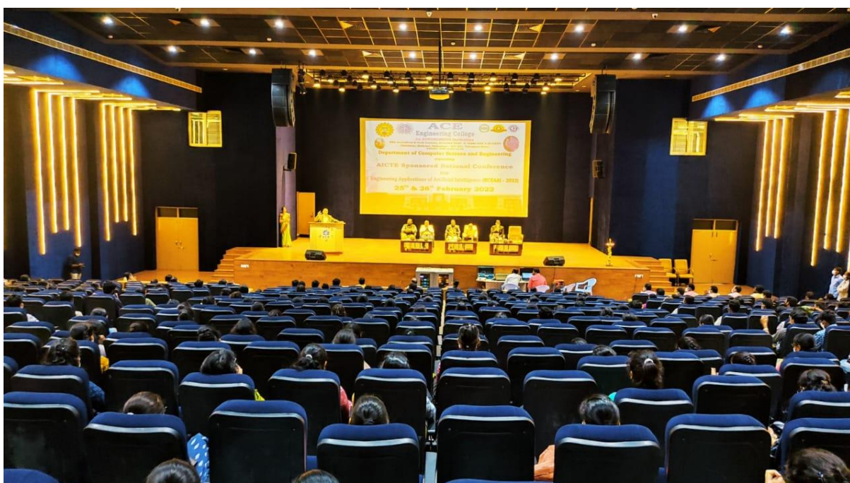
LED lights Inside Auditorium
